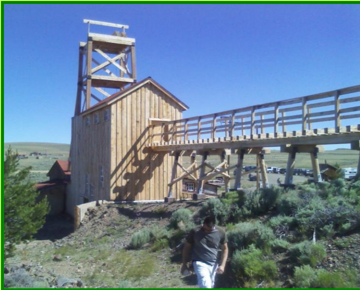
Carissa mine under construction.
